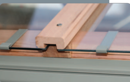
Glass on roof overhangs roof to prevent 'rot spots'
